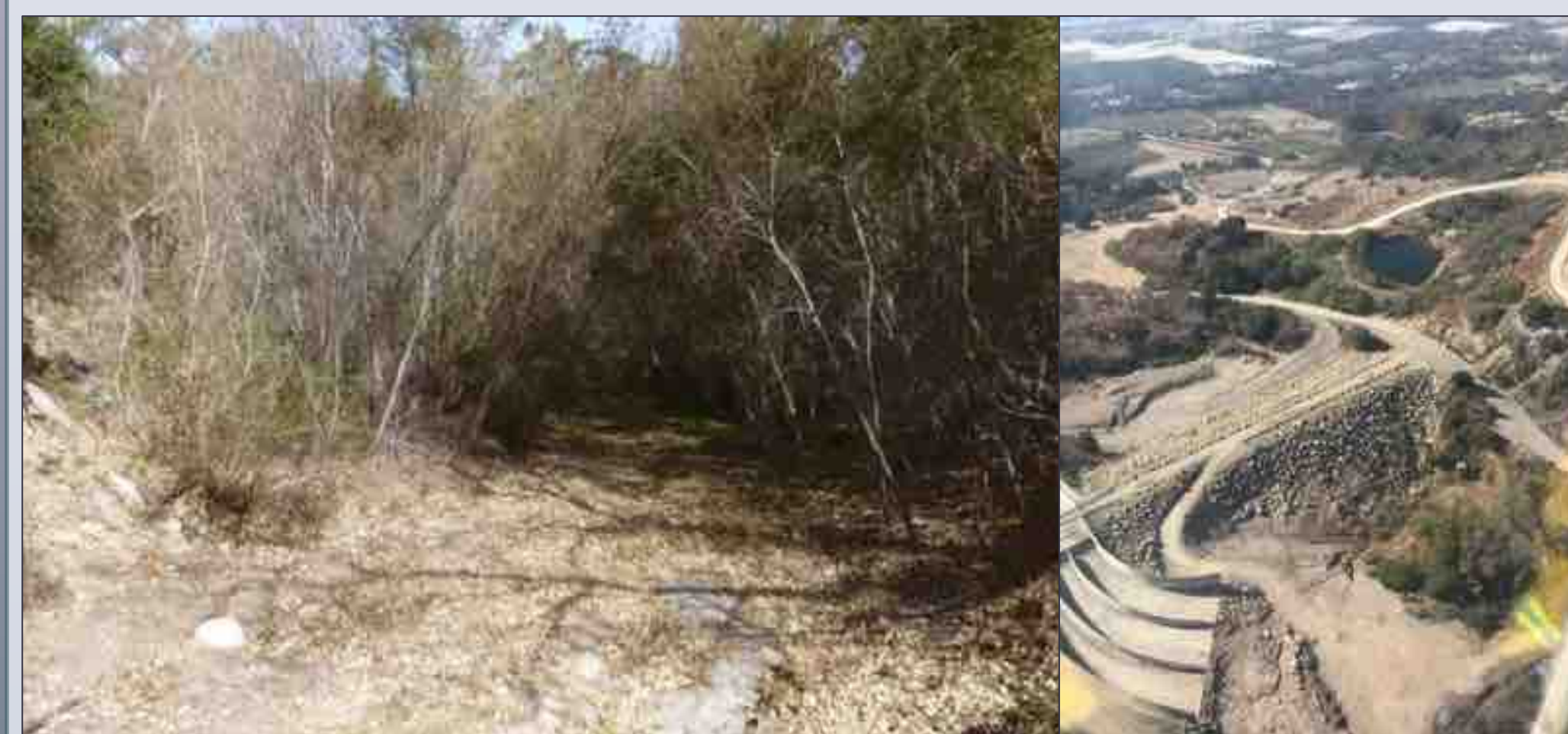
Figure. San Ysidro Creek Debris Basin (left) Santa Monica Debris Basin (right).
