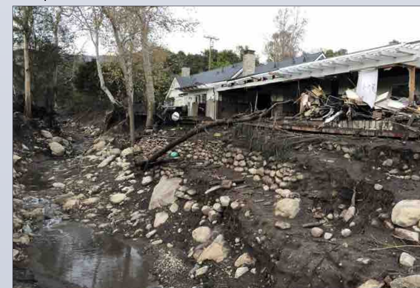
Figure. Damaged home in the immediate vicinity of the debris flow path in Montecito
