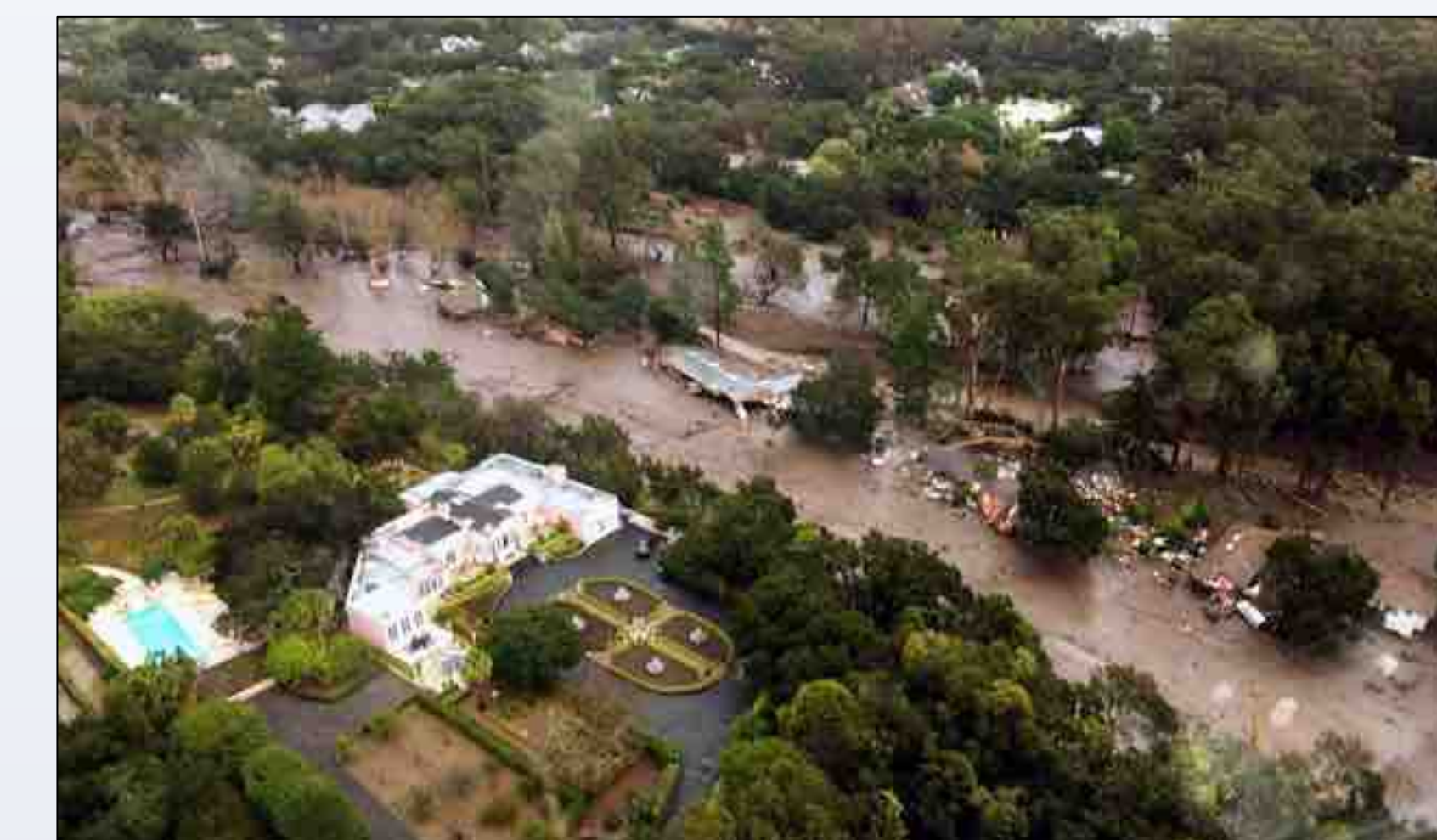
Figure 6. A residential area along San Ysidro Creek on Tuesday.
