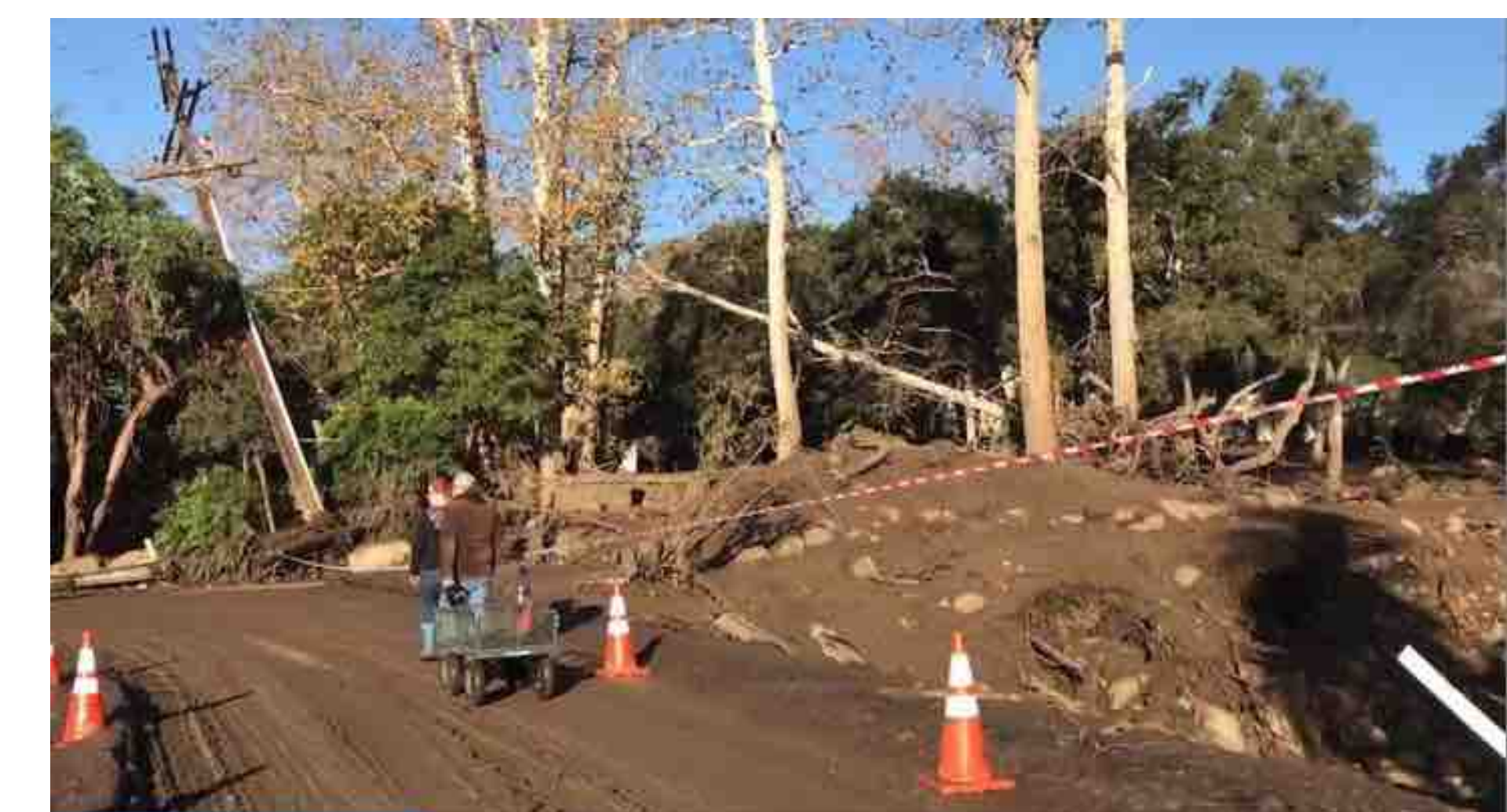
East Valley Road. Montecito, Marc Phillips slogged up and down East Valley Road Quote from local resident; "It looks like there was never a house there, but it was."
